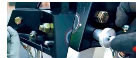
Pins Being Inserted into Holes atop Tripod
