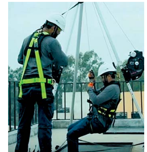
Worker Being Lowered into Confined Space
