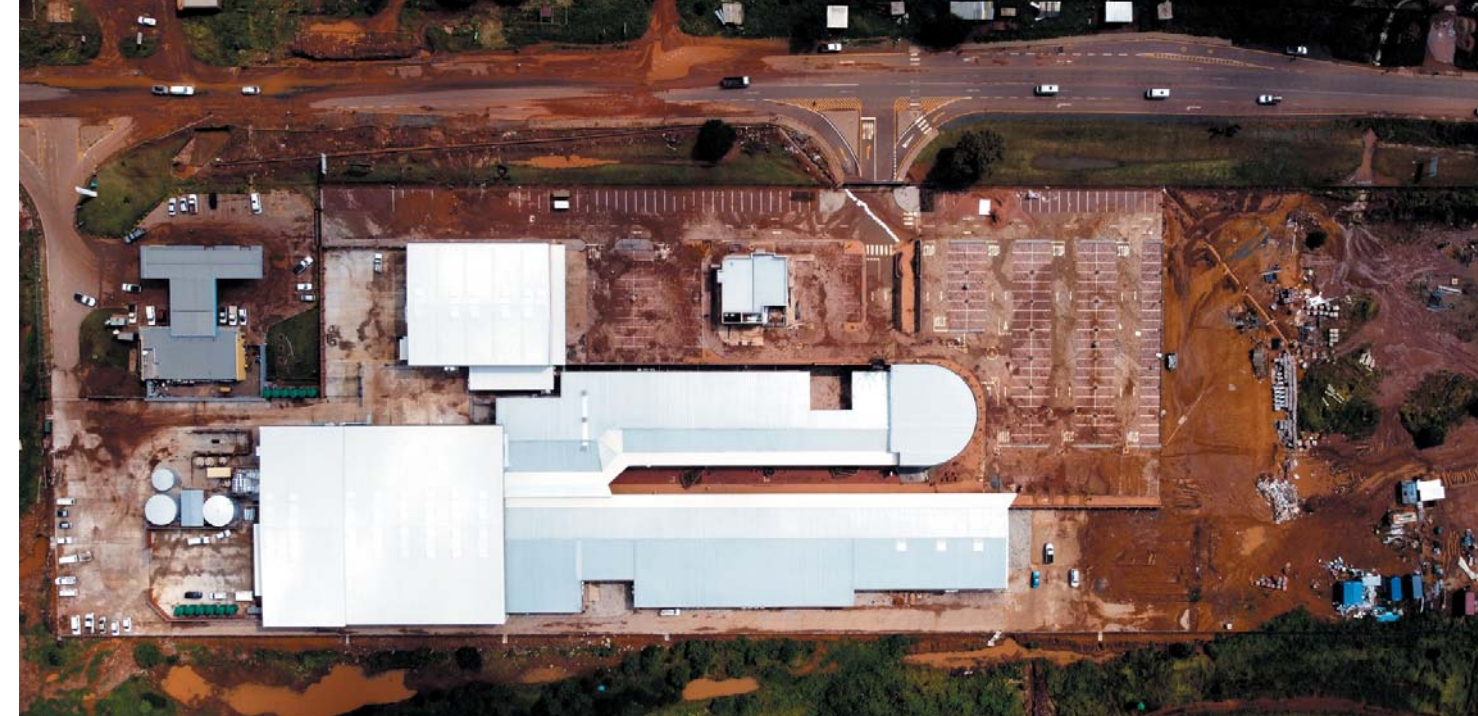
Aerial shot of the site during construction taken by Riscon
