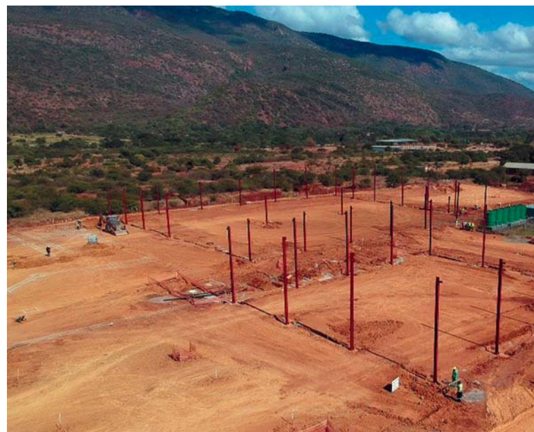
Construction started during 2019
