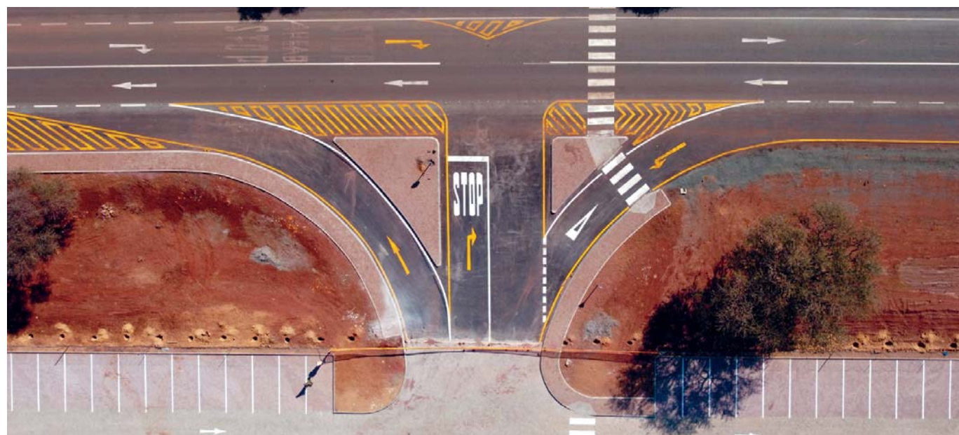
A major risk was accommodating and managing the passing traffic while constructing the road widenings and entrance to the development
